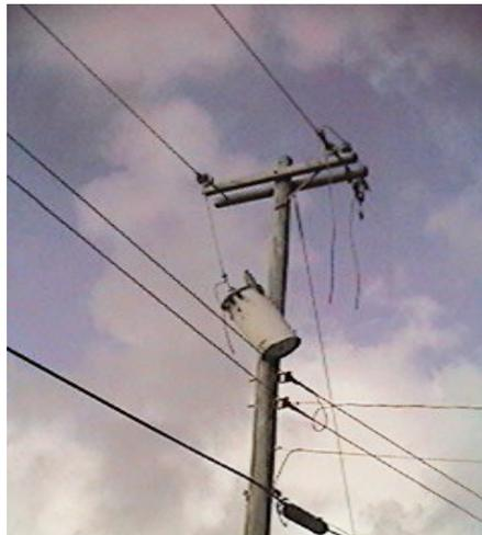
Figure 8 local transformer 4,000v-220v
